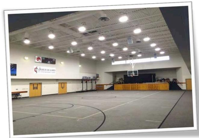
*StarTek 18" Lestra V1 fixtures replaced 250 metal halide fixtures in a gymnasium in Florida. Hanging height 24'.*
